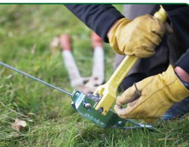
There is never a need to remove the underground Platipus cables, though by all means, cut the top cable out after 3 years to ensure it never comes into contact with the trunk of the tree as it grows. However, if fitted with an overhead guying system, after 2-3 years you can remove the overhead cables by simply cutting off the cable just below the ground at all three points, after which the rest will simply disassemble for disposal.
