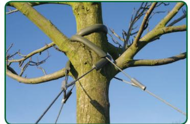
**If an overhead Platipus guying system is installed, you must inspect it at least once a year and slacken it off as necessary.**
